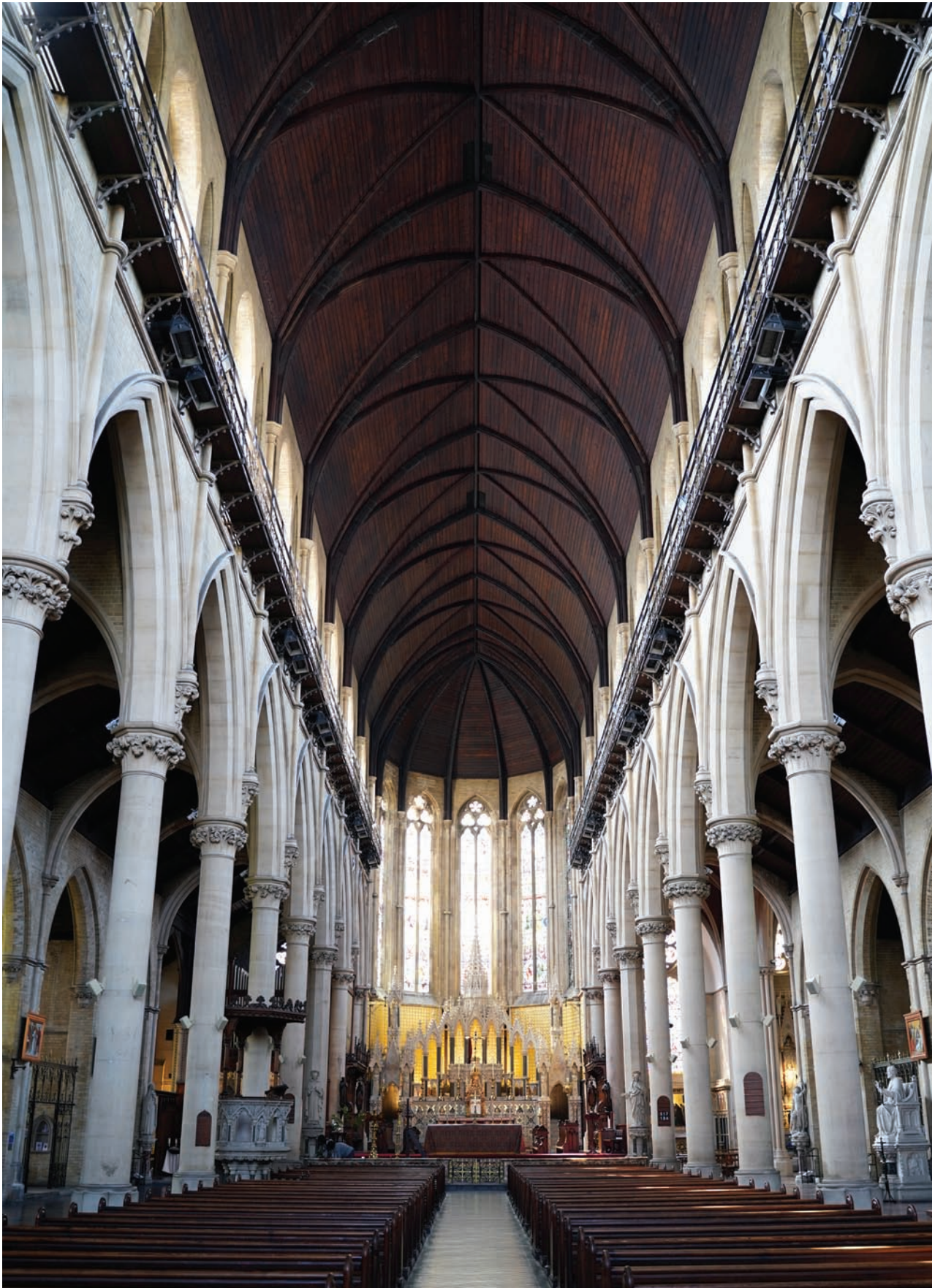
Fig 1. The priory church of Our Lady of the Rosary and St. Dominic, Southampton Road, Haverstock Hill, looking east. (photo: © Challe Hudson)
