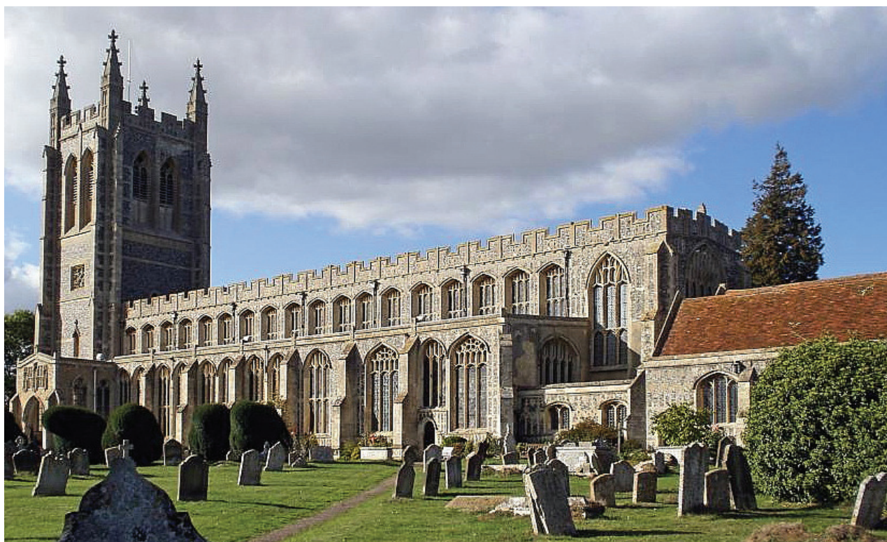
Fig 1. Holy Trinity church, Long Melford, Suffolk with the Martyn chapel at the east end of the south aisle, with a side door. (photo: © Martin Stuchfield)
