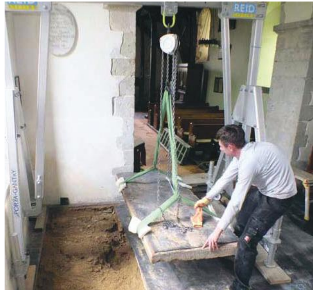
Lifting the Stapel brass and slab at Sutton. (photo: © Simon Nadin)
