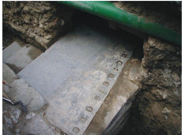
The top end of the slab
