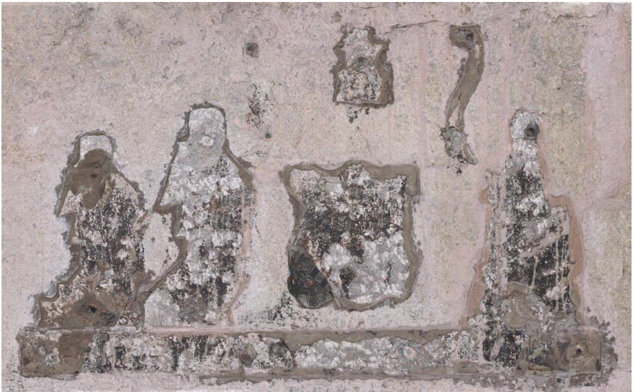
Fig. 3. The Purbeck slab of the Wylloughby brass (photographed on 25th October 2009) showing the surviving part of the achievement and the areas of cement
